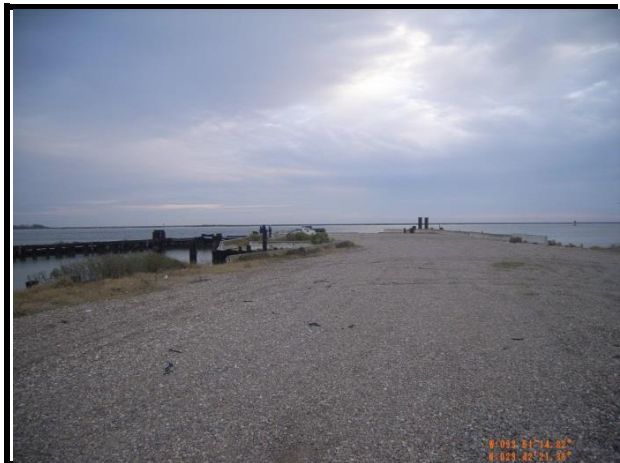
Dock on Texas Shoreline (Facing East)
