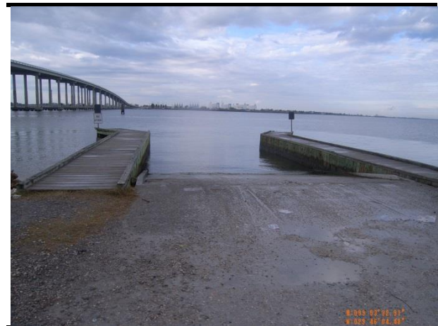
Public Launch Ramp in Louisiana, North of TX-82 (Facing West)
