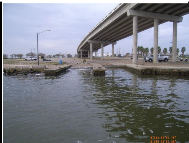
Public Launch Ramp in Texas, North & South of TX-82 (Facing West)
