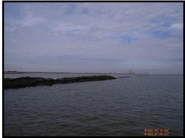
Texas Shoreline, Large Riprap Transitions to Submerged Small Riprap (Facing North)
