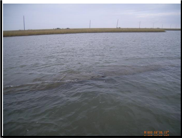
Texas Shoreline with Submerged Small Riprap (Facing West)
