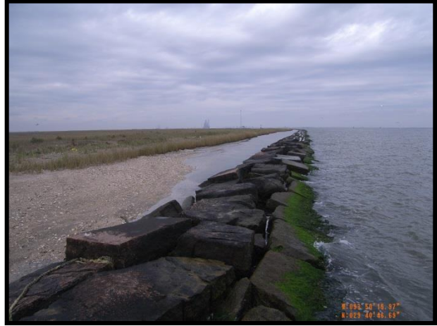
Texas Shoreline with Large Riprap and Marshes (Facing North)
