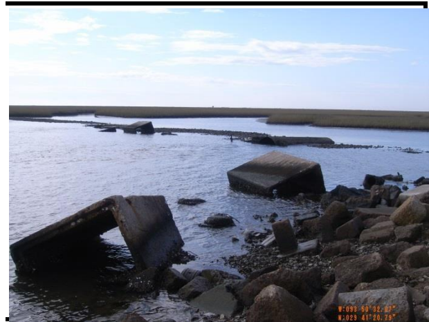
Texas Shoreline, Culvert Leading to Marshes (Facing West)
